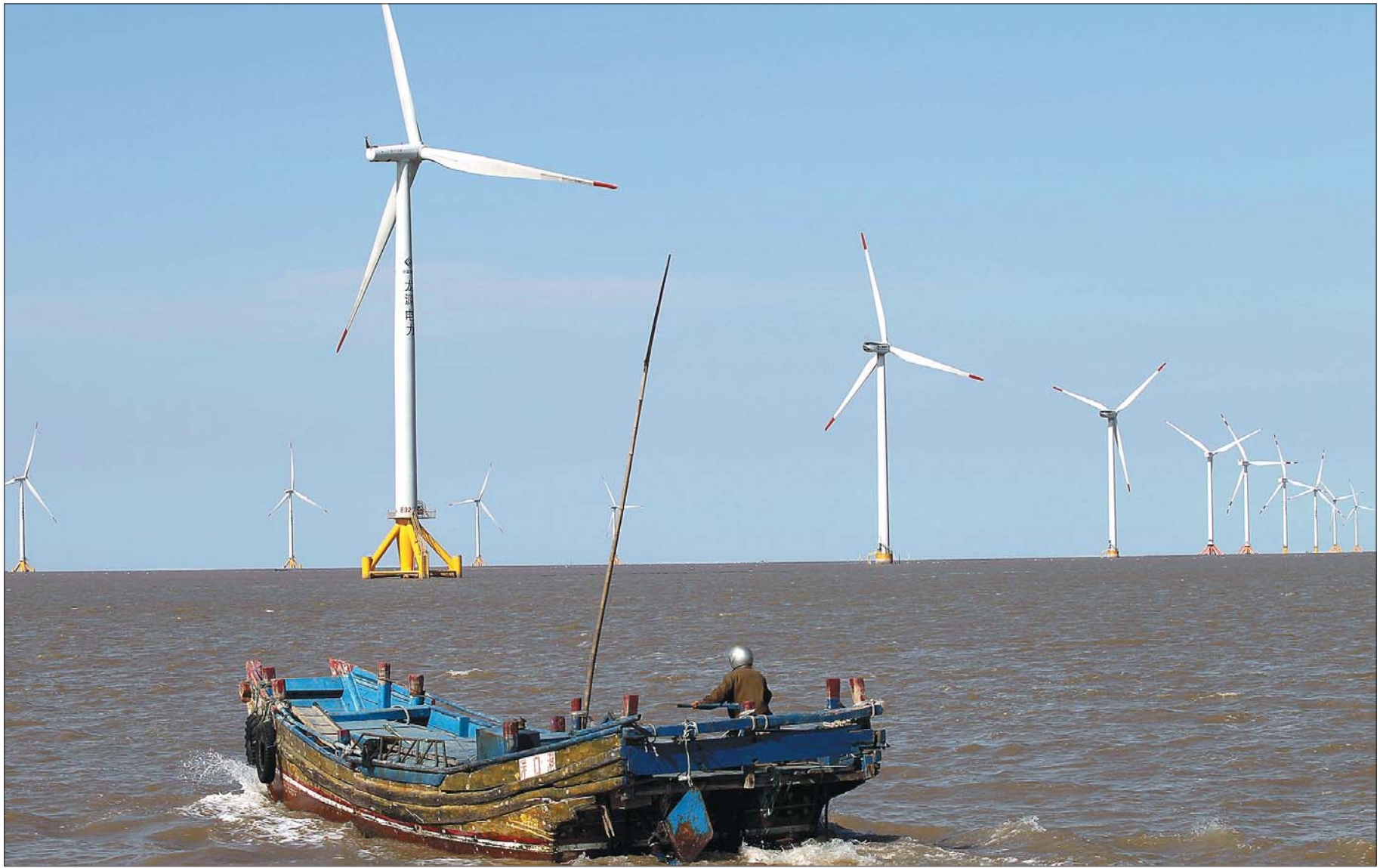
The fans at the 150-megawatt offshore wind power farm in Rudong county, Jiangsu province. China Longyuan Power Group completed the farm and put it into production in November.
